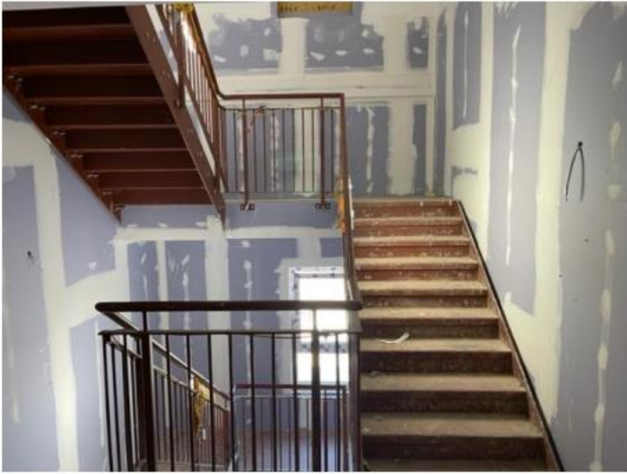
Stairwell Block C
