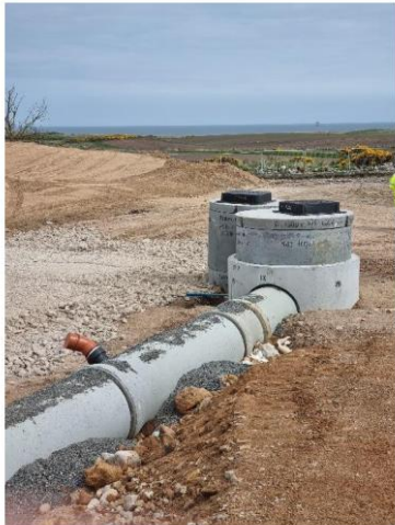
Photo 7 – Main drainage installed with typical connection visible at the pipe
