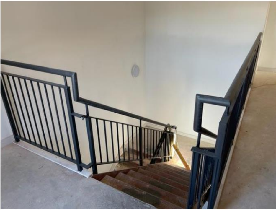
Stairwell Block B
